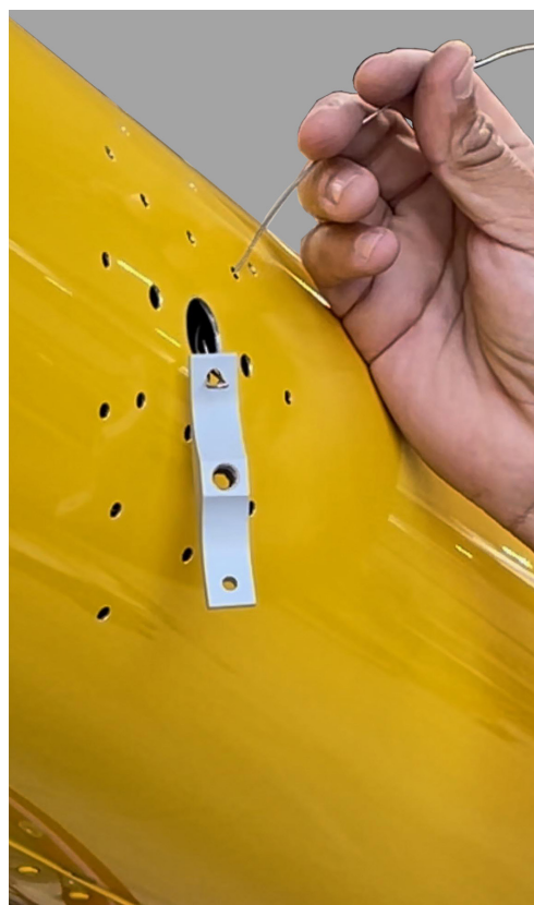
IMAGE 2 Installing F955-4 stiffener (RH side shown; LH side similar)
